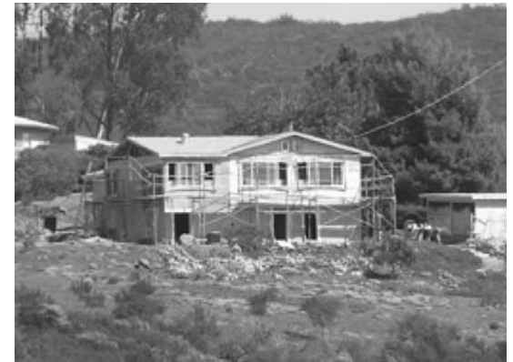
Wiltshire Home in Progress
